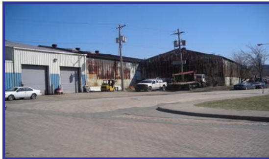
...and work at W & K Steel.
