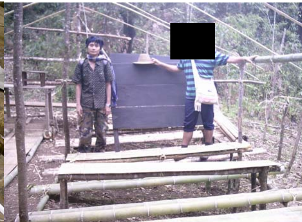
within days, the school is being rebuilt
